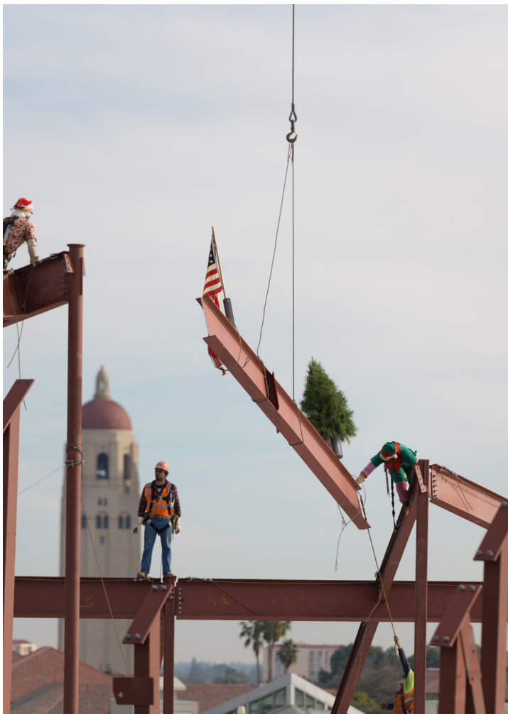
“Topping out” event for the new interdisciplinary research complex
